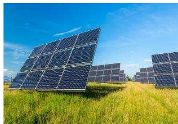
22MW solar farm in development (ENGIE & AMARENCO)
